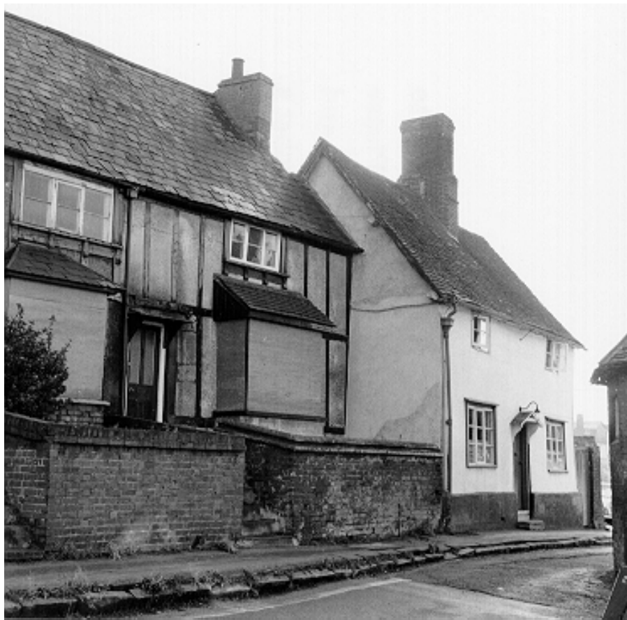
Wantage Grove Street - 1960s? - Nos.34, 32 (renovated 1975), and 30 (16th C, was "Rose & Crown"). (Surveyed J Garnish 1982) (st070.jpg)
